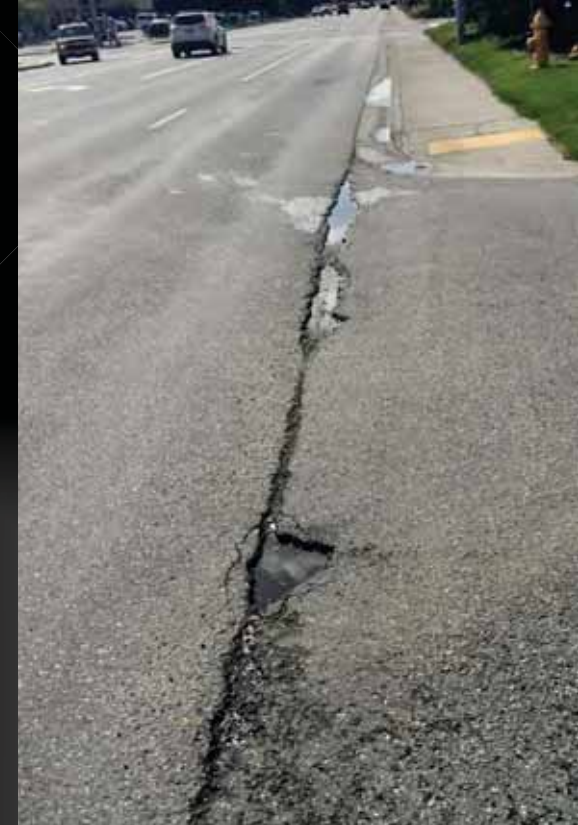
Road Surface Deterioration
